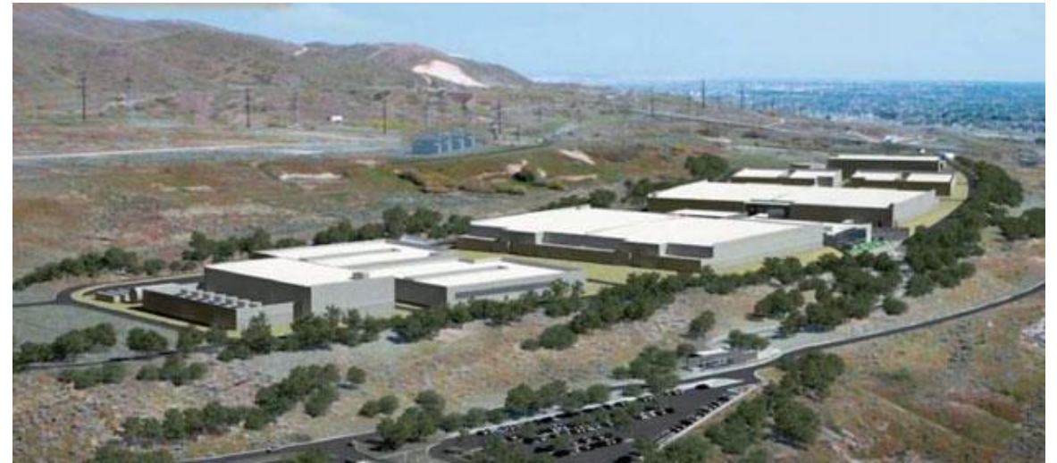
Bumblehive - NSA Utah Data Center, Bluffdale Utah
